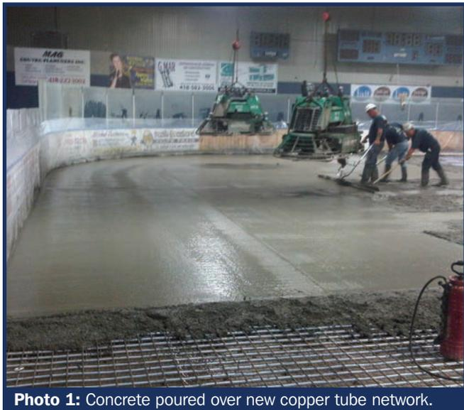
**Photo 1:** Concrete poured over new copper tube network.
