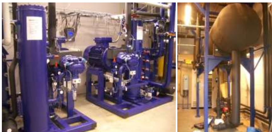
Figure 6. The Backavallen ice rink in Sweden with CO 2 as secondary refrigerant in copper tubes.
